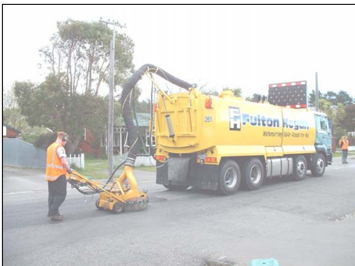
Figure 2. Water supply and vacuum recovery system
