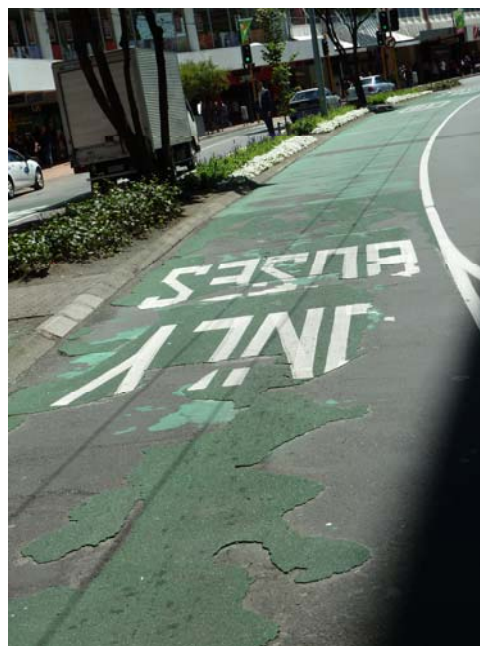
Figure 2: Surfacing delamination
