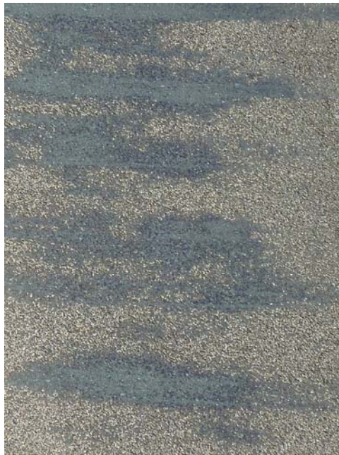
Figure 1: Calcined bauxite chip loss
