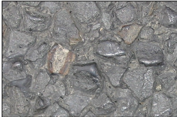
Figure 2. Polished and rubber/binder coated aggregate tips
