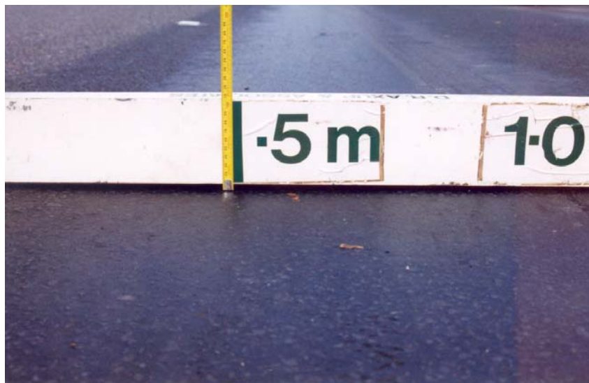
Figure 5: Rutting and flushing in the left hand lane
