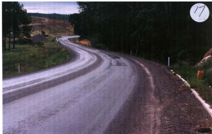
Figure 2: The D'Aguilar Highway, Queensland. Dry, as shown, 0.7. Wet 0.16
