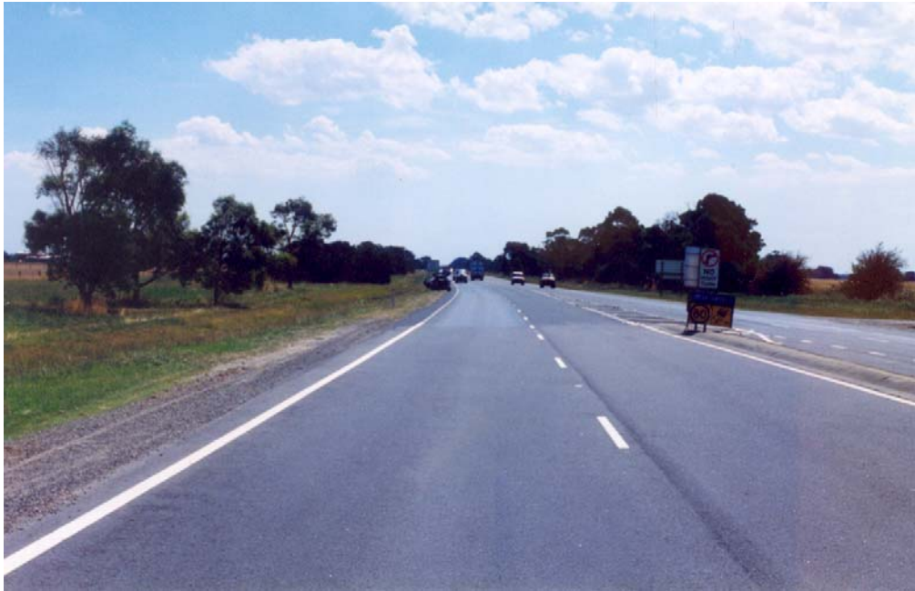
Figure 4: The section of road involved. Note the change in surface and the difference between the left and right lanes beyond the change.
