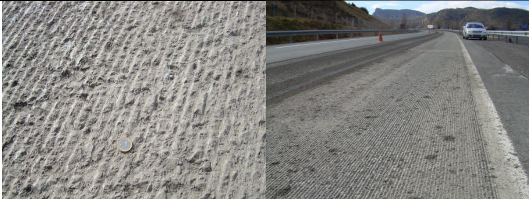
Figure 11. Final appearance after microgrinding
