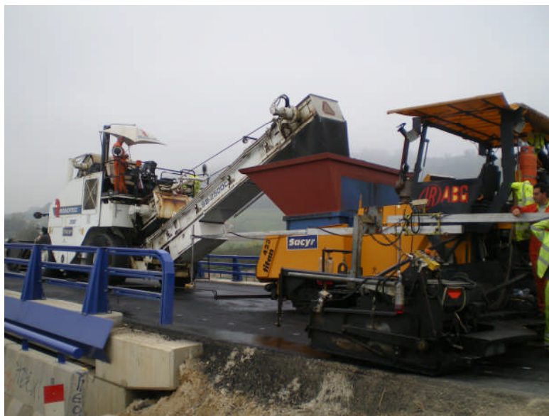
Figure 2. Roadtec SB-2500 Shuttle Buggy MTV
