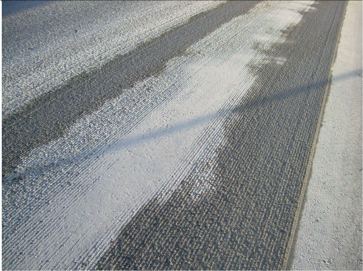
Figure 14. Right-hand rut to which microgrinding was not applied.
