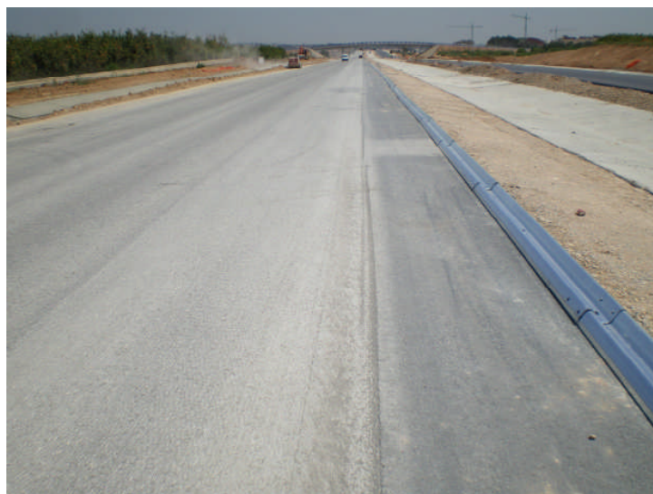
Figure 3. Final result of grinding to improve roughness.
