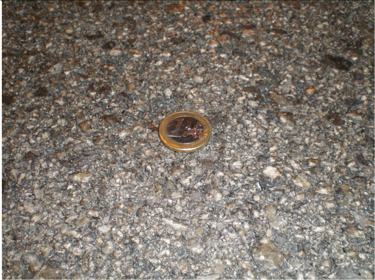
Figure 8. Detail of improvement in micro- and macro-texture after blasting.
