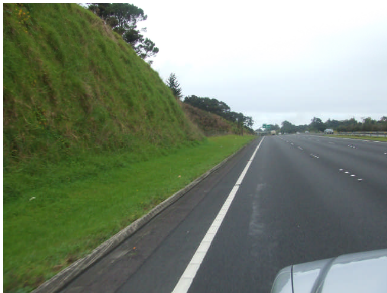
Figure 10: Unprotected Slope on existing motorway
