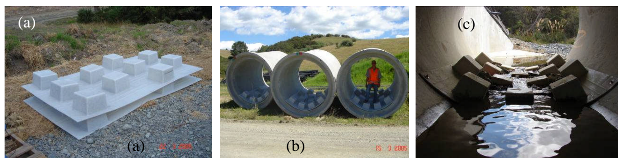
Figure 4: Plastic fish spoiler sheets: a) as manufactured; b) placed in culverts and c) installed in culvert as riffles with matrix of natural materials.
