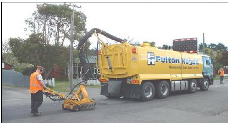
Figure 4: Ultra High Pressure Watercutter in Operation.
