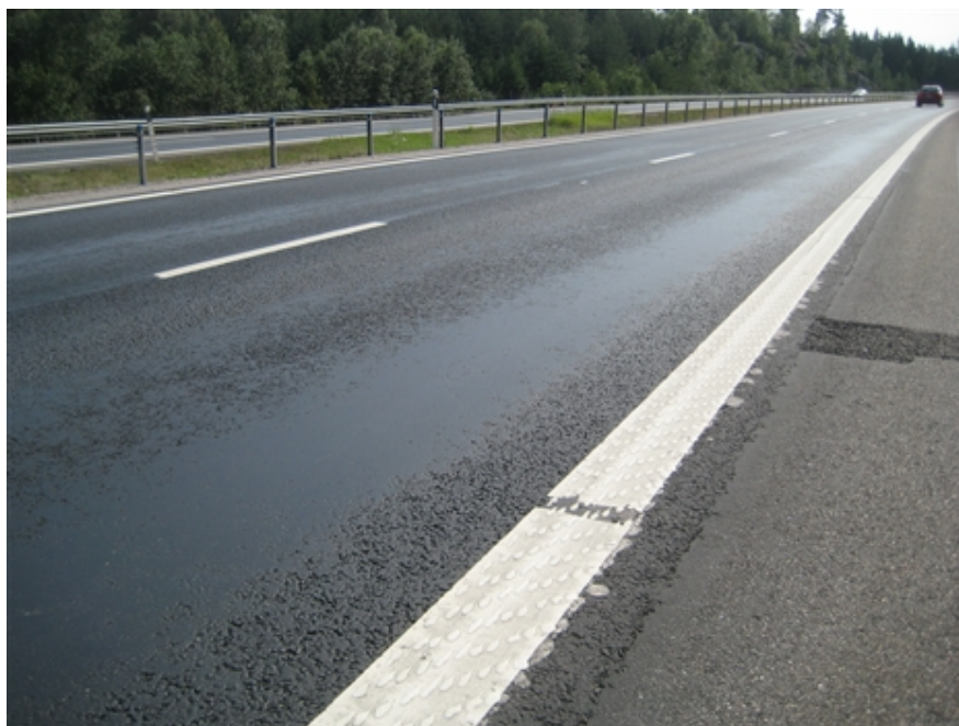
Figure 2: New paved "bleeding" pavement
