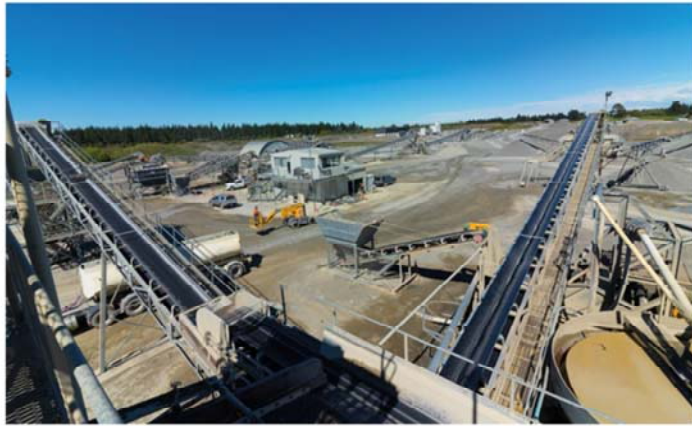
Miners Road quarry Christchurch Source: Quarry and Mining Magazine
