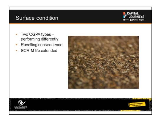
While we have achieved the aim of SCRIM compliance, we have found as a consequence of the removal of the upper surface, we have accelerated the rate of ravelling, therefore failure of the integrity of the OGPA. This is most likely due to cracking of the bitumen during the milling process.
