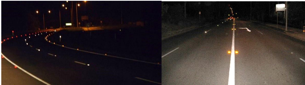
Figure 1: RRPMS at reduced frequency at Caboolture-Bribie Island Road and Samford Sub-arterial Road
