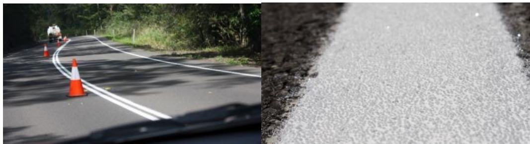
Figure 2: Cold applied plastic at Beaudesert-Beenleigh Road and Nambour-Mapleton Road
